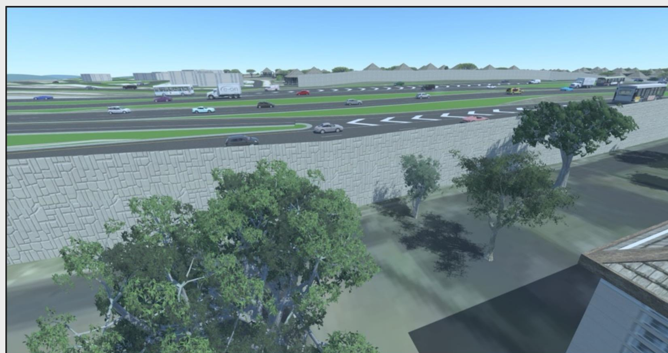
B) Birdseye – Back of Noise Wall
