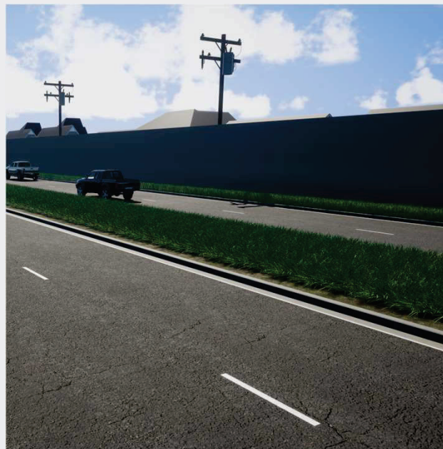
Street view front of wall
