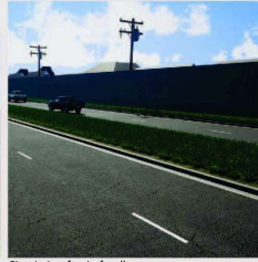
Street view front of wall
