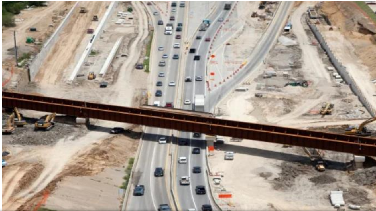
North Tarrant Expressway, Tarrant County, TX
