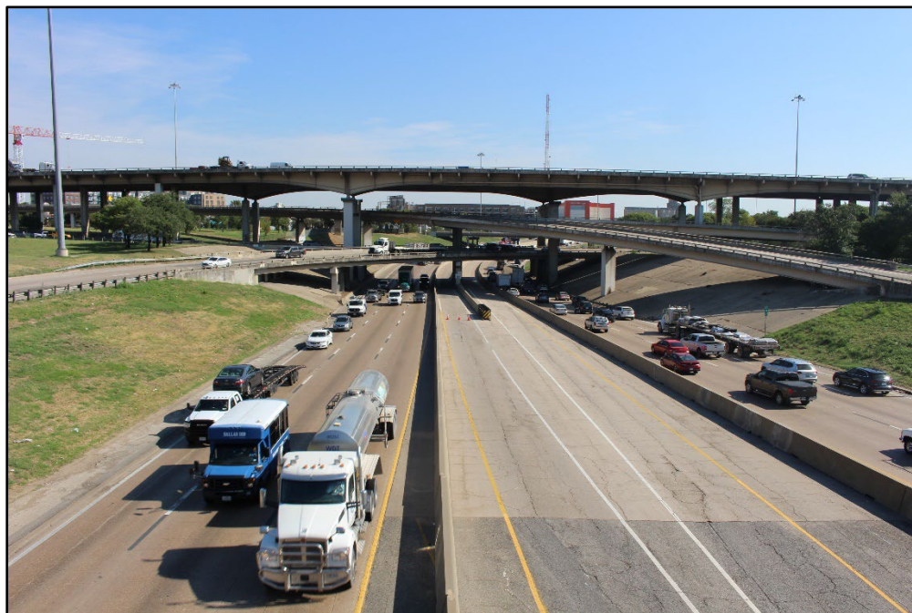
Photo 24 – Looking east along I-30 at its system interchange with I-345 / I-45 from the S. Good Latimer Expy. bridge. The interchange is proposed to be reconstructed.
