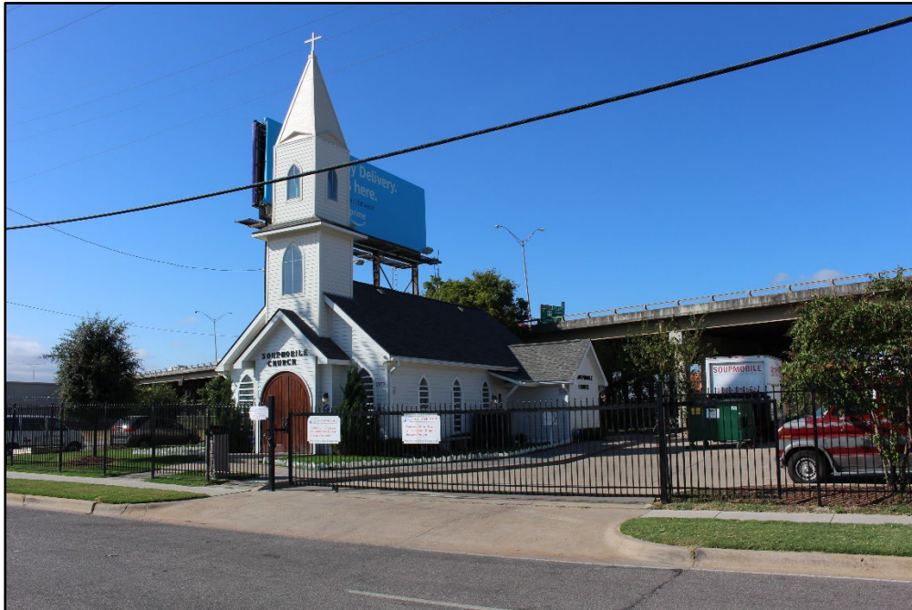
Photo 30 – Looking southwest at SoupMobile Church located at 2423 S. Good Latimer Expy.
