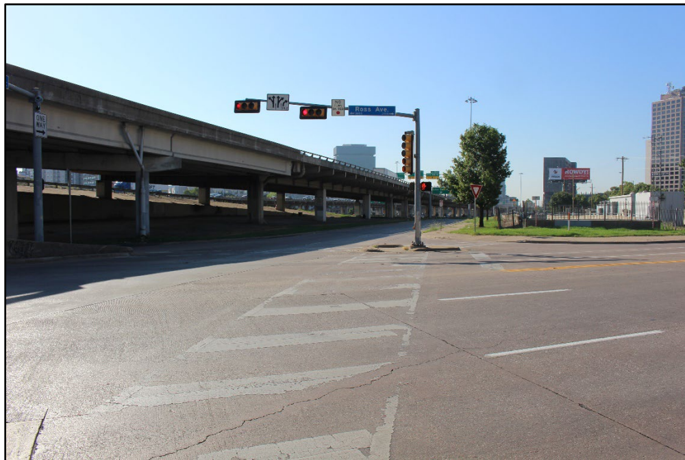
Photo 8 – Looking south along the I-345 facility at Ross Ave.
