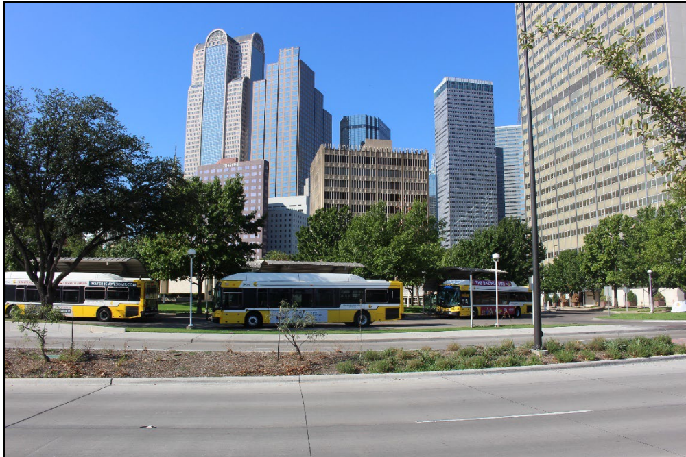
Photo 16 – Looking west at the Central Business District East Transfer Station.
