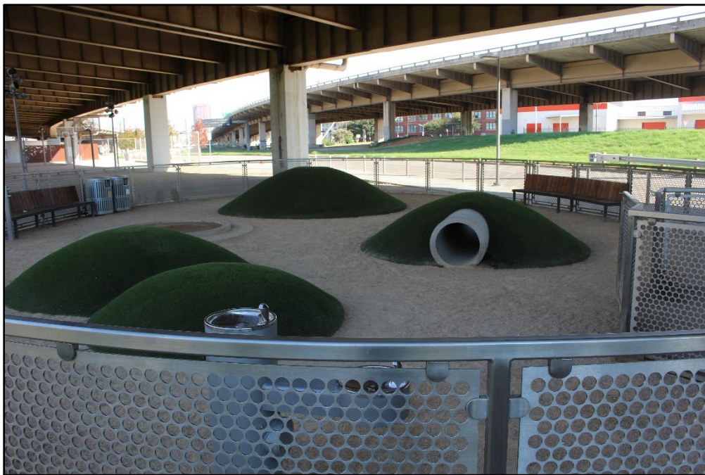
Photo 18 – Looking northeast at the dog park within Carpenter Park located underneath the existing facility that would be removed as a result of the Build Alternative.
