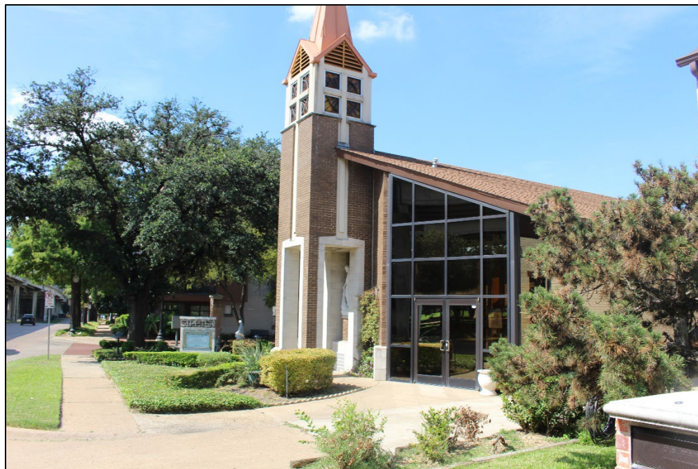
Photo 6 – Looking southeast at St. Peter the Apostle Catholic Church located at 2907 Woodall Rogers Fwy.
