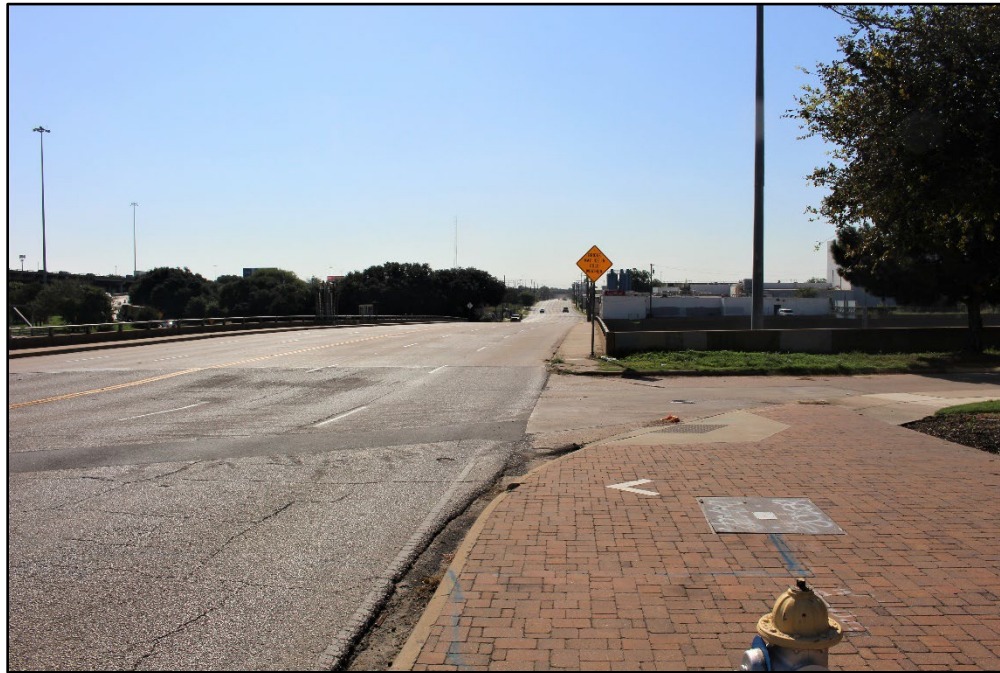
Photo 23 – Looking south along S. Good Latimer Expy. as it crosses I-30.
