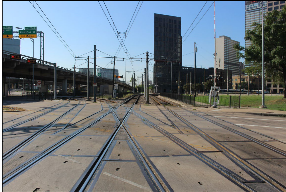
Photo 13 – Looking south at the existing DART at-grade crossing of N. Good Latimer Expy.
