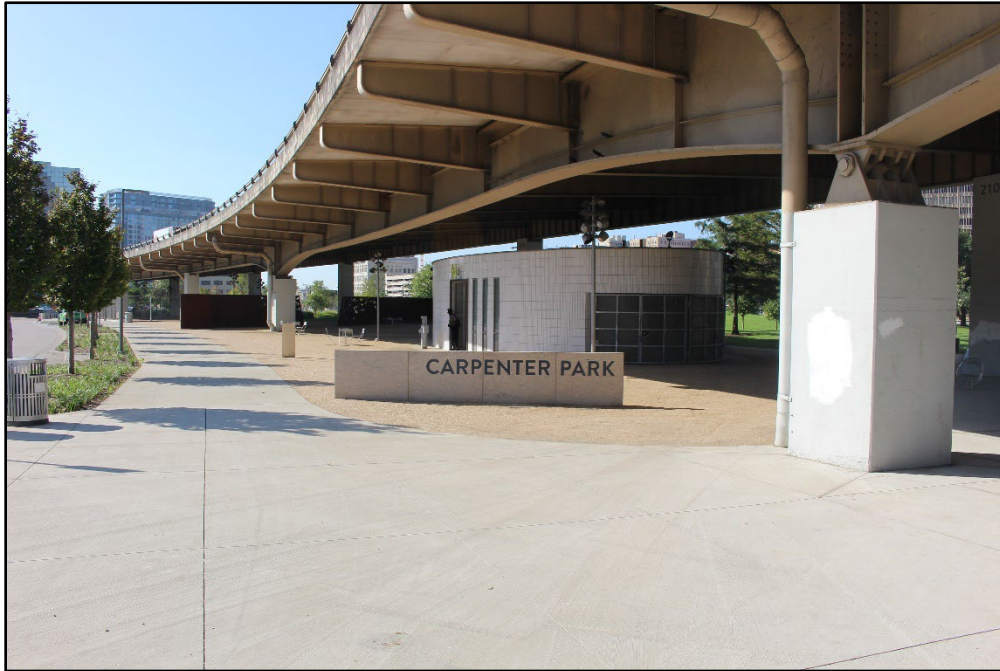
Photo 15 – Looking south at Carpenter Park located at 2201 Pacific Ave. The park is partially underneath the existing I-345 facility and within TxDOT ROW.
